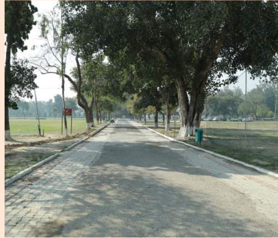
"Paving the Way to Progress: Widening Our School's Roads with Pavers!"
